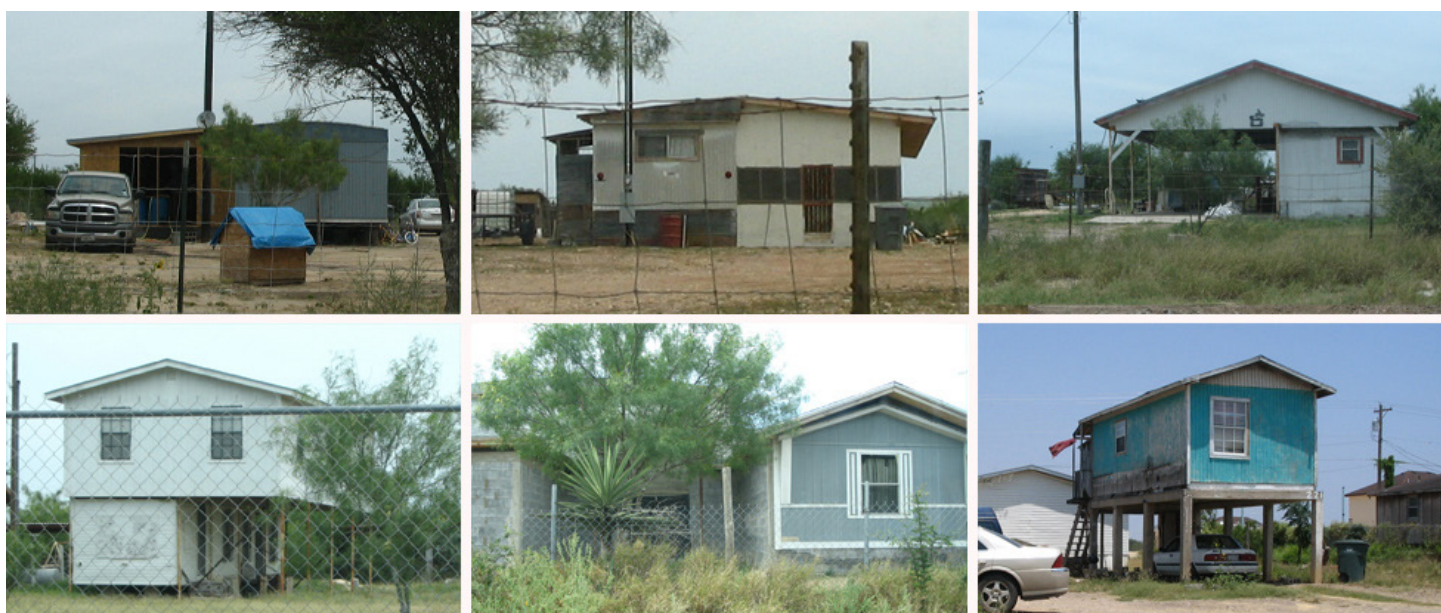
Figure 4. Manufactured mobile houses modified to enlarge or improve the house structure
